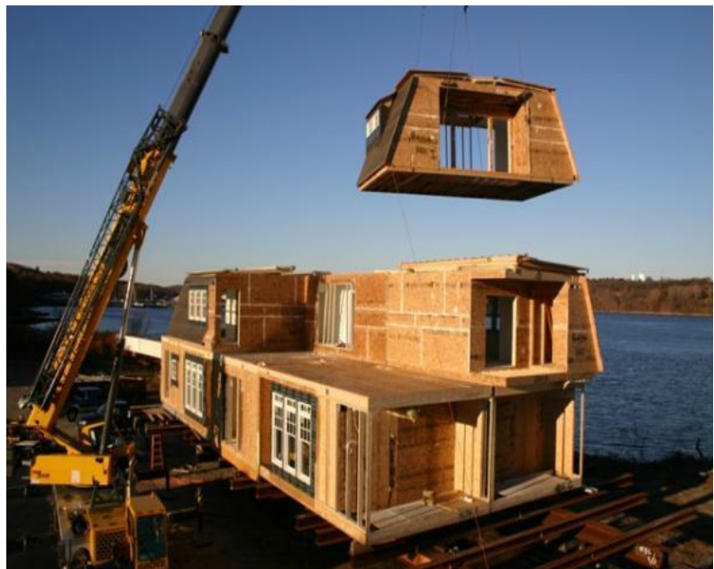
Fig 43: Construction of Modular House
