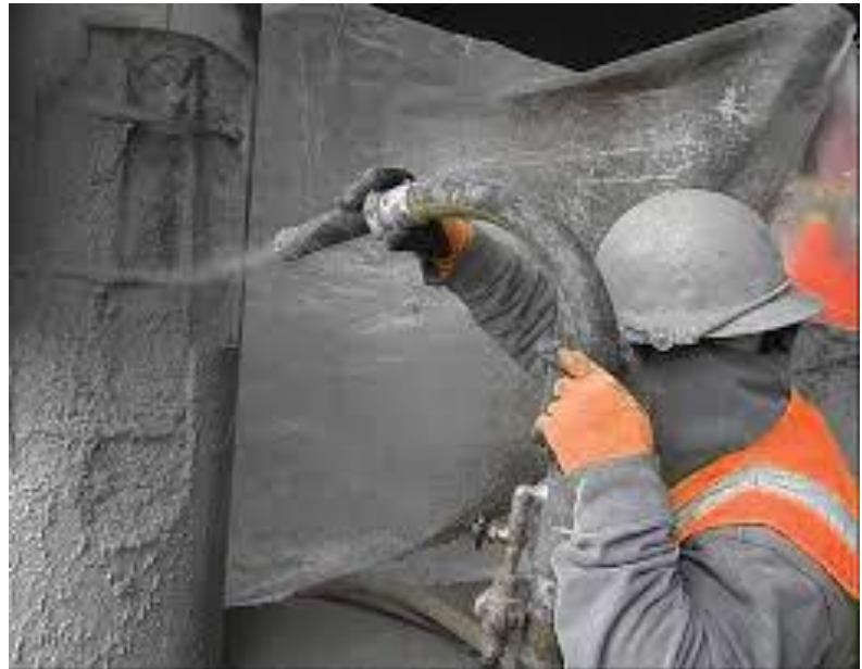
Fig 51: Repair and protect deteriorated RCC
